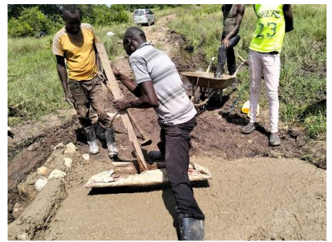
Finishing off the culvert
