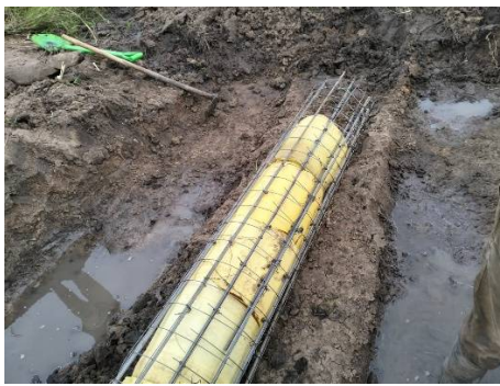
Creating our own culvert
